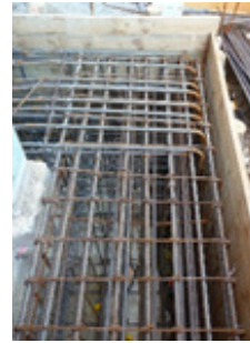
Figure 2. A view of the reinforcing of the new foundation beam with an existing corner column to the left.
