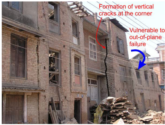
Figure 4b. Typical URM construction in Nikosera: formation of vertical cracks at corners which resulted in separation of cross wall from main wall
