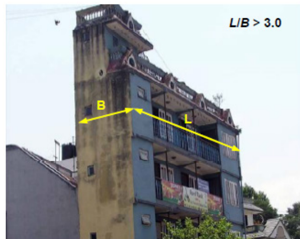
Fig. 7. An example of RC building with upper storeys supported on long cantilever slab or beam, and (b) a building with very large length to width ratio ( L/B )
