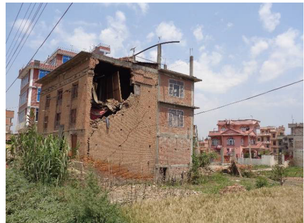
Figure 5b. URM buildings failures in Nikosera: combined in-plane and out-of-plane failure of the wall
