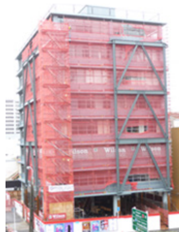
Figure 3. The new steel eccentrically braced frames have just been craned into position and now need to be strongly attached to each floor diaphragm at beam level.
