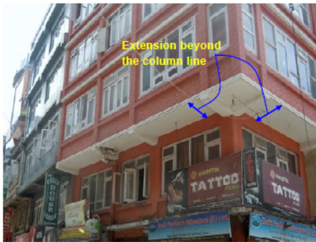
Fig. 7. An example of RC building with upper storeys supported on long cantilever slab or beam, and (b) a building with very large length to width ratio ( L/B )
