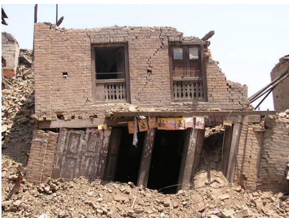
Figure 5a. URM buildings failures in Nikosera: collapse of three storey unreinforced masonry building
