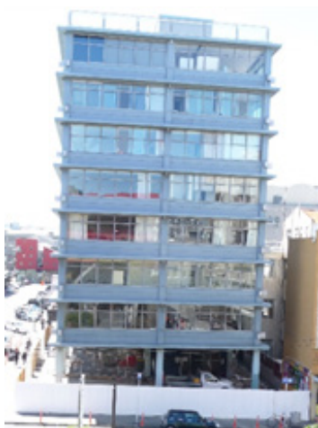
Figure 1. Elevation of the building being retrofitted. Note weak columns and strong perimeter beams.
