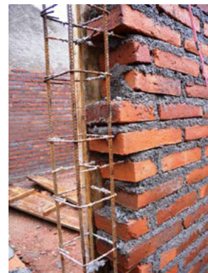
(b) a toothed wall-to-tie-column interface
