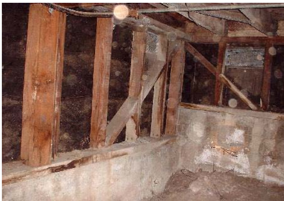
Figure 246 Cripple Wall before Retrofit Source: http://www.boltusa.com
