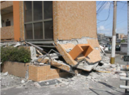
Figure 18: Failure of the southern wall due to the soft storey collapse
