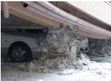
Figure 7: Crushed column in south frame
