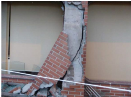
Figure 12: Shear failure in a column
