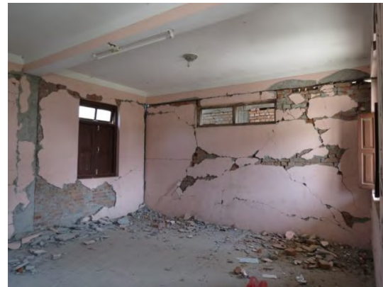
Figure 23: Severe damage to infill walls due to diagonal and shear sliding crack at mid-height of walls in a school building at Sankhu (photo and annotations: Hemant Kaushik)
