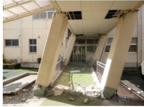
Figure 14: Story drift in the east corridor
