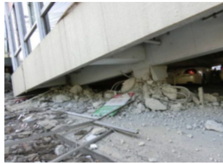
Figure 20: Southern columns crushed in the soft storey
