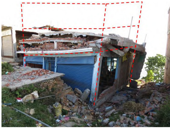
Figure 24: Poor seismic design and detailing in combination with poor geometric configuration resulted in severe damage in RC frame buildings with masonry infill walls: (a) collapse of a four-story building at Irkhu, (b) failure of beam-column joints in the same building, (c) rupture of reinforcing bars in first-story columns of the same building (photos and annotations: Hemant Kausbik)
