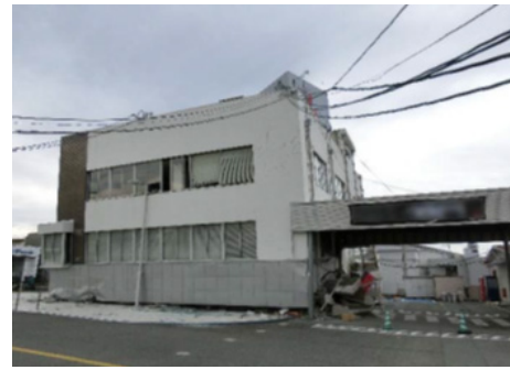
Figure 9: Southern view. The whole ground floor has been lost.
