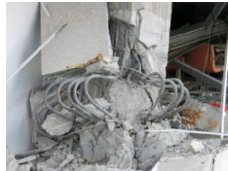
Figure 10: A crushed column
