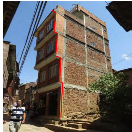
Figure 26: Large overhangs in one direction at building in Dhulikhel (photo and annotations: Hemant Kausbik)
