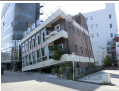
Figure 19: The soft storey collapse from the north-east
