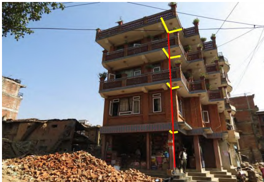
Figure 25: Large overhangs in both directions at building in Sankhu (photo and annotations: Hemant Kausbik)
