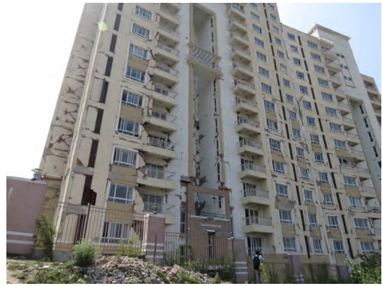
Figure 22: Severe damage to infill walls along both in-plane and out-of-plane directions in the high-rise apartment building at Dhapasi (photo and annotations: Hemant Kaushik)
