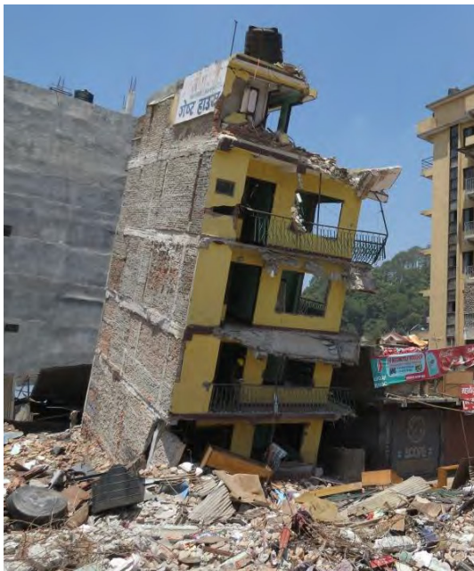
Figure 21: Damage sustained by RC frame buildings with masonry infills with different heights: (a) three-storey building in Chautara, and, (b) six-storey building in Balaju, (photos: Hemant Kaushik)
