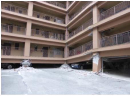
Figure 6: Soft ground floor or 1st storey collapse in the north east frame
