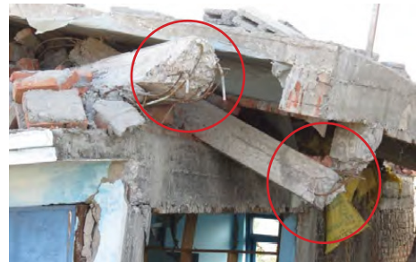
Figure 24: Poor seismic design and detailing in combination with poor geometric configuration resulted in severe damage in RC frame buildings with masonry infill walls: (a) collapse of a four-story building at Irkhu, (b) failure of beam-column joints in the same building, (c) rupture of reinforcing bars in first-story columns of the same building (photos and annotations: Hemant Kausbik)
