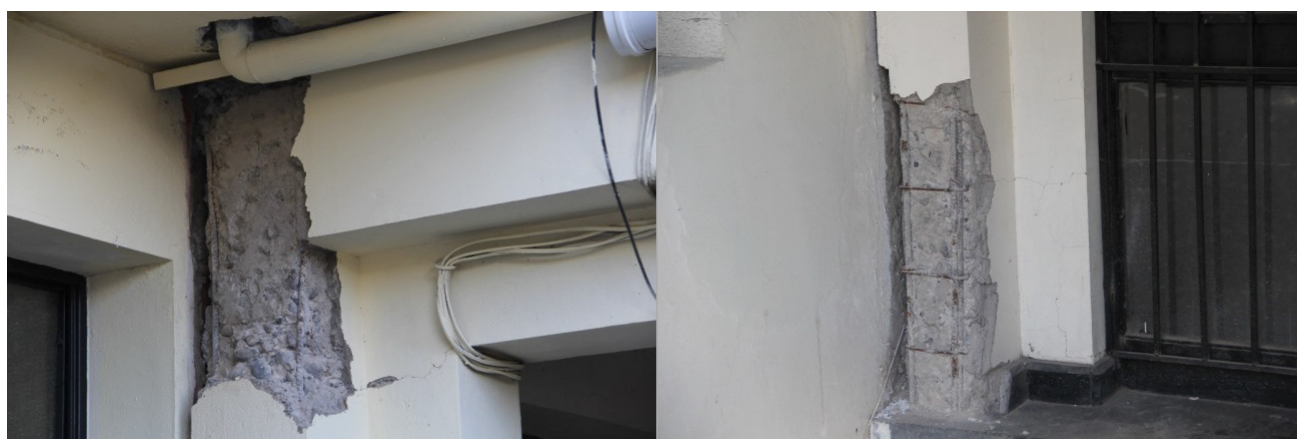
Figure 6: Spalling of concrete was observed in structural elements in the hospital of Illapel (Photos: Claudio Fernández).
