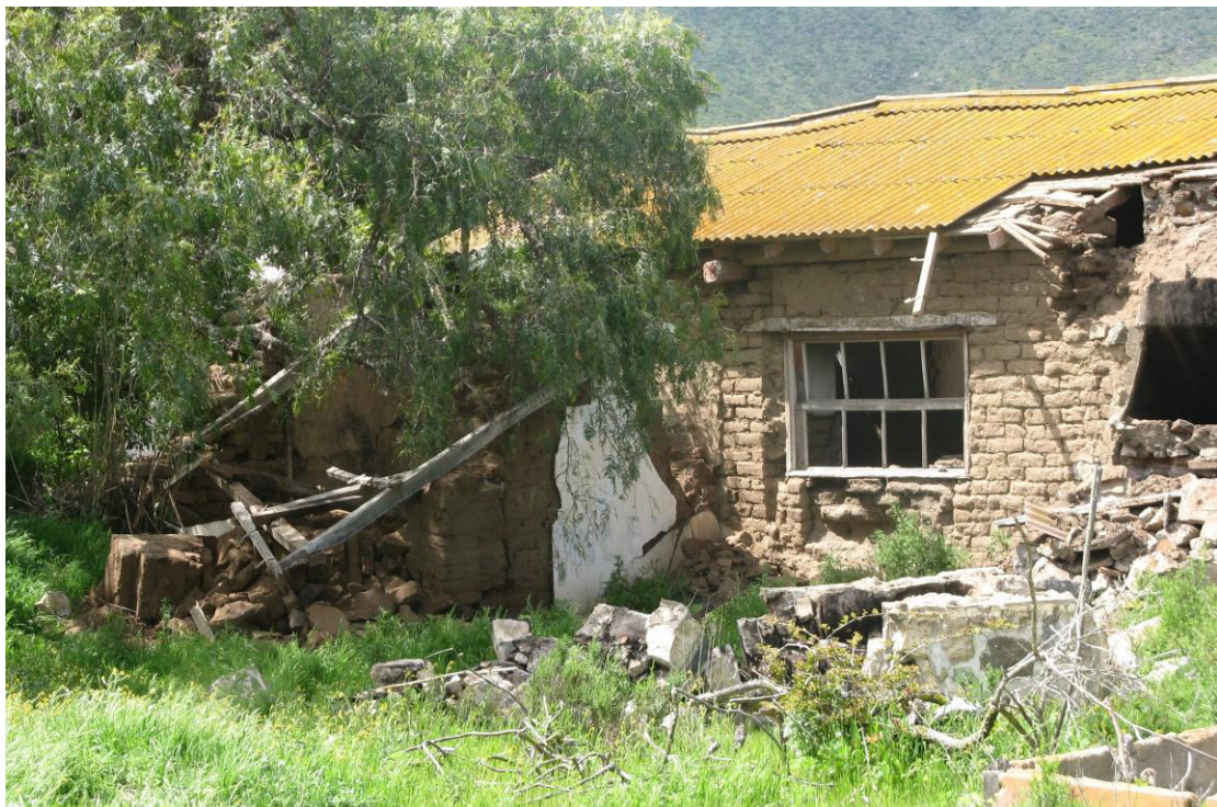
Figure 9: Damage caused by the strong ground motion in adobe structures. Communa de Canla Baja, km 283 at 5 route.
