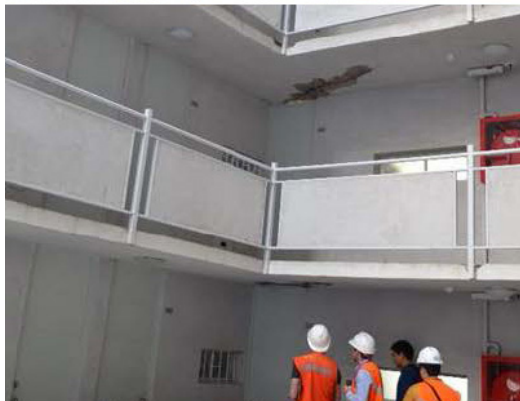
Figure 8: Damage concentrated in specific areas of the slabs of the Puerto Babia condominium. La Herradura, Coquimbo.
