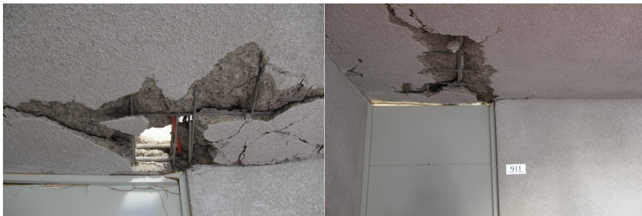
Figure 5: Structural damage in the slabs of a RC building in La Herradura, in the city of Coquimbo (Photos: Claudio Fernández).
