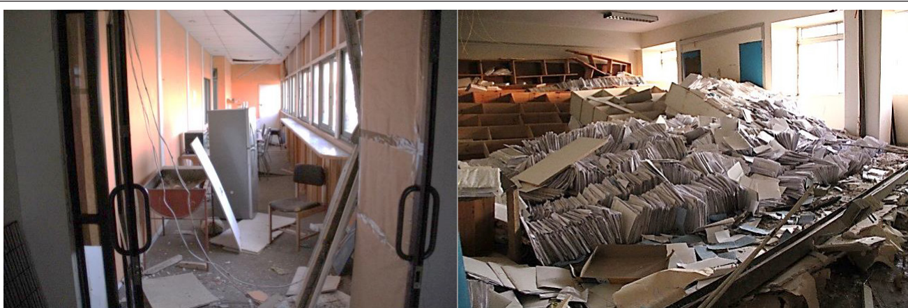
Figure 4: Non-structural damage decreased the capacity of providing healthcare services in the Coquimbo hospital (left). Some of the hardcopies of the medical records, without digital backup, were lost in the region (right) (Photos: Claudio Fernández).
