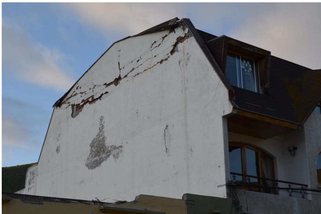
Figure 7: Masonry structures affected exclusively by strong ground motion. Illapel.
