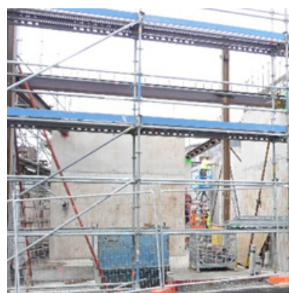
Figure 3. Two shear walls near one corner of the building. Other shear walls are placed around the plan to provide strength in both plan orthogonal directions and with reasonable symmetry to avoid excessive torsion.
