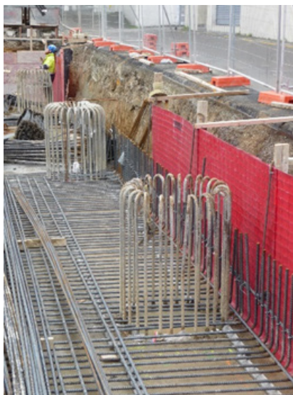
Figure 1. Reinforcement for the bored piles projects above the soffit of the raft slab.
