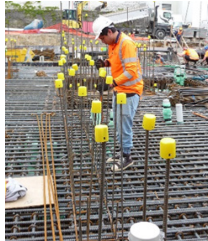
Figure 2. A worker adjusts reinforcing steel in the raft foundation. The vertical bars are the starters for the shear walls.
