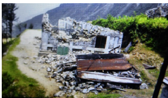
Fig. 7 Complete collapse of retrofitted school building in Rasuwa
