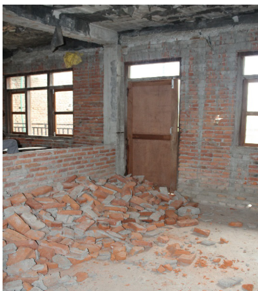
Fig. 6 School building 101-1 experiencing only moderate shaking deemed unsafe.
