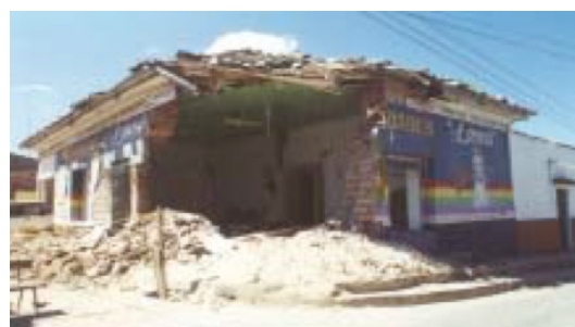
Figure 3. Total collapse of adobe walls
