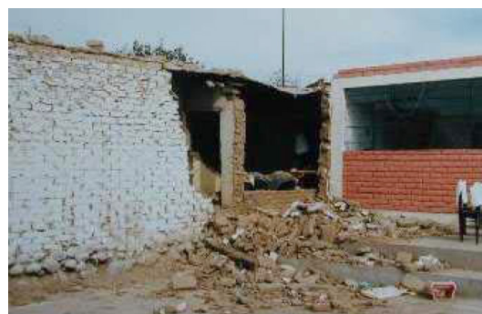
Figure 2. Out-of-plane wall collapse
