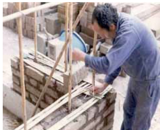
Figure 6. Vertical and horizontal reinforcement
