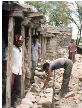
Figure 15. Construction of an uncoursed random rubble stone wall in Maharashtra, India
