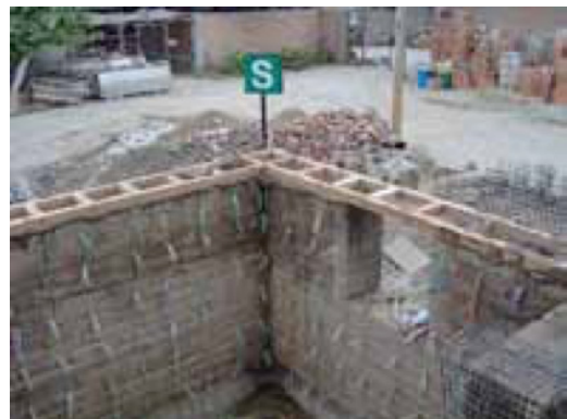
Figure 5. A wooden ring beam
