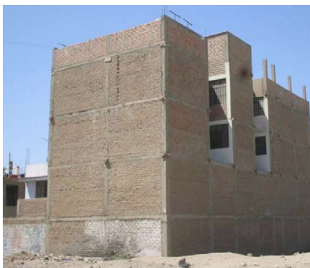
Figure 8. Performance of a confined masonry building in the 2007 Pisco, Peru earthquake
