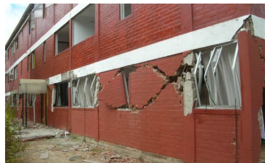
Figure 9. In-plane shear failure of poorly confined masonry walls in the 2010 Maule, Chile Earthquake
