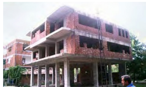
Figure 13. Infill walls influence the behaviour of a RC frame: if the infills are absent at the ground floor level this modifies the load path, which is detrimental to earthquake performance causing a soft storey
