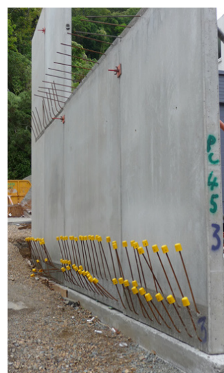
Figure 3. Reinforcement at the base of a precast panel to tie it into the floor slab.
