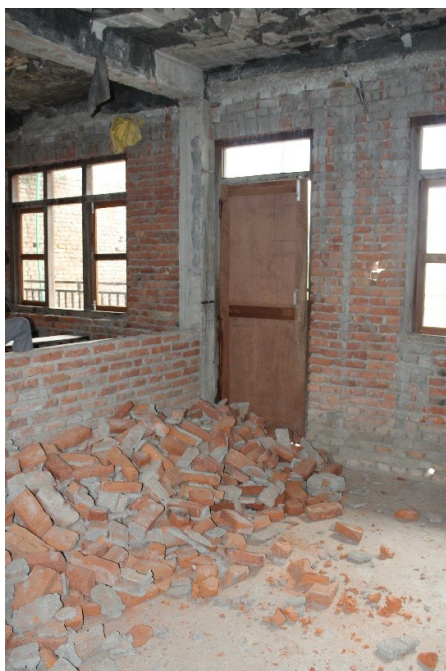
Figure 5. School building 101-1, which experienced only moderate shaking in Bhaktapur, was deemed unsafe for school use because unreinforced partition walls separated from the reinforced concrete frame and became unstable. Damage to unreinforced partition or infill walls can injure or kill students and block exits. The safety of these walls is routinely ignored by engineers and communities alike.
