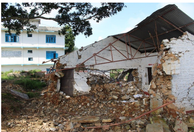
Figure 6. This teaching resource centre on school grounds was built with stone and mud mortar. The masons employed earthquake-safety measures, such as a reinforced concrete lintel band and vertical reinforcement in the walls. However, even with these measures, the heavy shaking in Sindhupalchowk caused the stone building to collapse swiftly and completely. It may be difficult to rebuild safe schools out of this brittle material unless alternative technologies are developed, tested and extensive mason training and strict oversight are feasible during construction.
