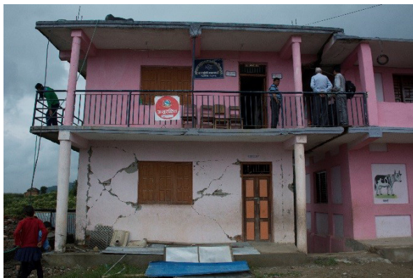
Figure 4. At a school in Kathmandu, two school buildings on the same sight performed very differently. The building on the left, a reinforced concrete frame structure with brick infill walls, was moderately damaged and received a red tag. Its frame joints and infill walls will need to be repaired before the building can be reused for classrooms. The building on the right, an adobe and stone masonry structure, was recently retrofitted with stitch banding. It was undamaged and immediately able to be reopened, despite being made of a weaker building material. The retrofit proved to be successful.
