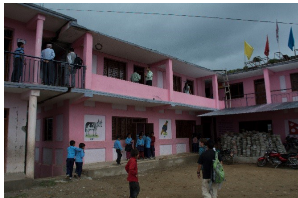
Figure 4. At a school in Kathmandu, two school buildings on the same sight performed very differently. The building on the left, a reinforced concrete frame structure with brick infill walls, was moderately damaged and received a red tag. Its frame joints and infill walls will need to be repaired before the building can be reused for classrooms. The building on the right, an adobe and stone masonry structure, was recently retrofitted with stitch banding. It was undamaged and immediately able to be reopened, despite being made of a weaker building material. The retrofit proved to be successful.
