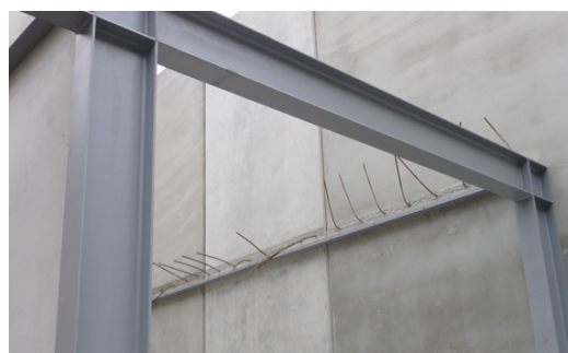
Figure 2. Steel frame and panel to suspended floor connection detail.
