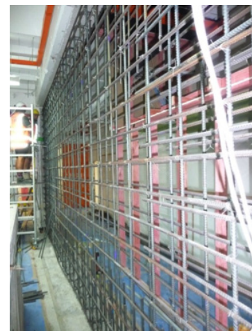
Figure 2. A completed reinforcing cage ready to be enclosed by formwork prior to casting the concrete.
