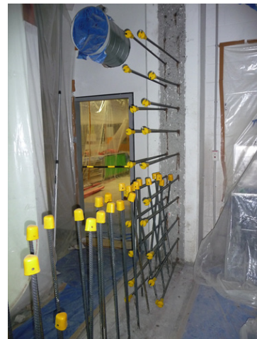
Figure 1. Horizontal and vertical reinforcing starter bars have been grouted into the existing beams and columns of the moment frame.
