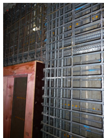
Figure 3. Additional reinforcing steel is required to trim openings and to ensure adequate force paths within the infill.
