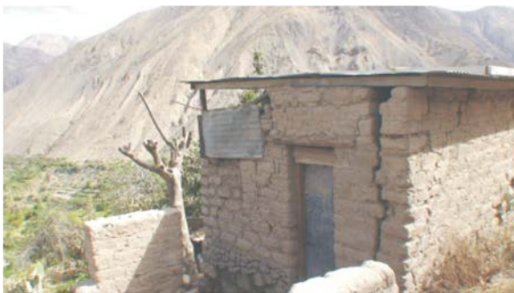
Figure 4. Non-engineered adobe house in Peru showing vertical crack and separation of orthogonal walls owing to out-of plane forces
