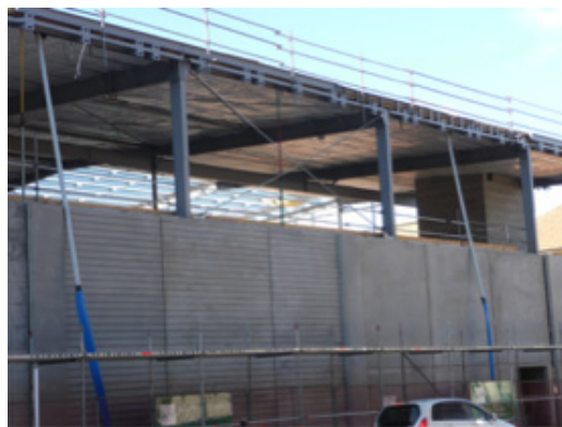
Figure 1. View of the ground floor precast concrete panels and the steel first floor framing.
