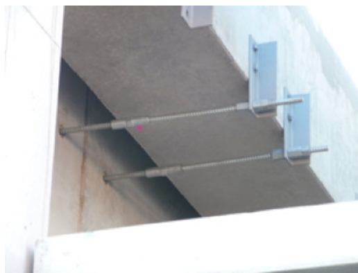
Figure 2. Precast concrete panel to reinforced concrete beam connection.
