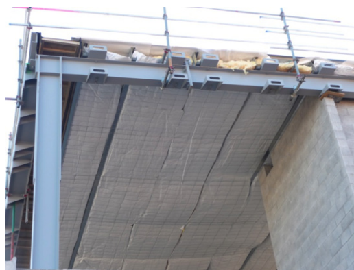
Figure 3. The first floor steel moment frame with steel brackets to facilitate connection of precast concrete panels.
