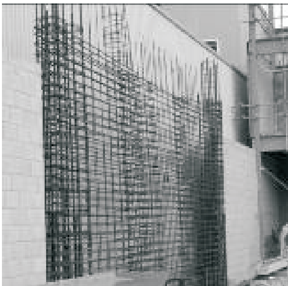
Fig. 1 RC shear wall reinforcement between reinforced concrete masonry walls.
