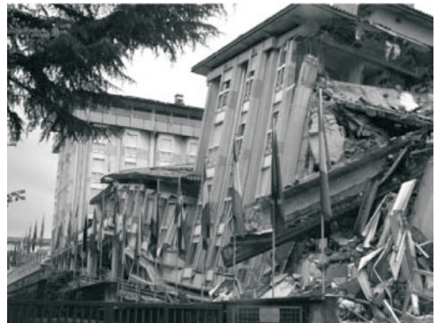
Fig. 8 Collapse of part of the Duca D'Abruzzi Hotel caused by a softstorey mechanism. The far part of the building was saved by a seismic separation joint.
