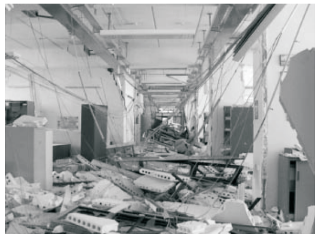
Fig. 9 The interior of the City Planning Offices in L'Aquila. Note that the building exterior has very minor detectable damage.
