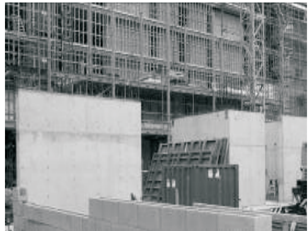
Fig. 3 Internal RC shear walls acting in the longitudinal direction.
