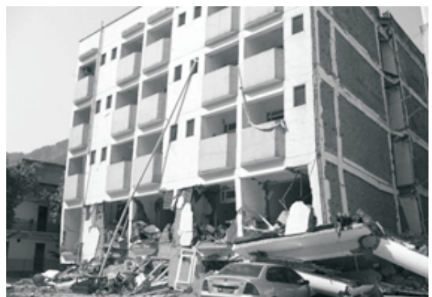
Fig 11: Soft-story collapse, Hanwang Hospital.
