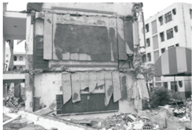
Fig 10: URM wall and RC floor plank collapse, Juyuan Middle School.
