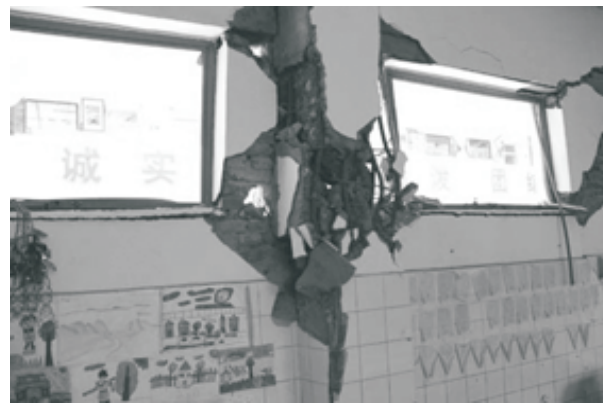
Fig 12: Captive column failure, Hanwang High School.
