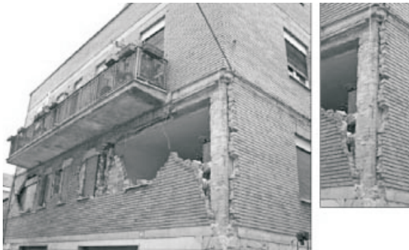
Fig. 7 Typical damage to infill walls.
