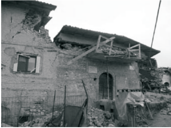
Fig. 6 Collapse of a masonry building in Tempera with concrete ring beam retrofit.
