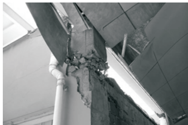
Figure 13: Column flexural damage, Mianzhu Experimental
