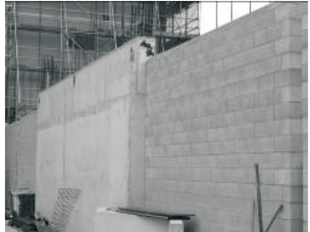
Fig. 2 Poured ground floor level transverse shear wall.
