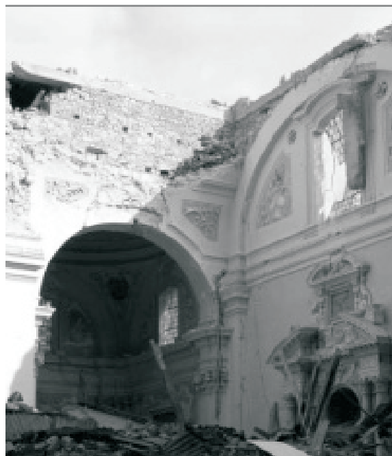
Fig. 5 Roof and cupola collapse in the Santa Maria di Collemaggio Abbey in L'Aquila. The reinforced concrete ring beam did not prevent the collapse of the cupola.
