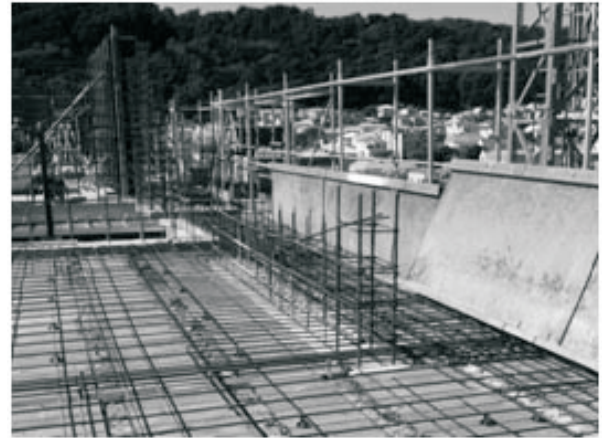
Fig. 2 Precast ribs and permanent timber infills with diaphragm reinforcement awaiting topping concrete pour. Note the band of heavy diaphragm reinforcement to the right.
