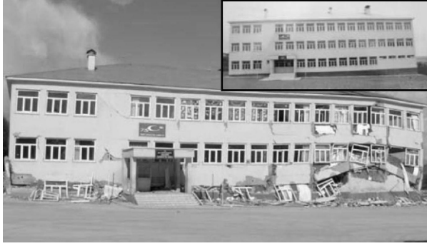
Fig. 5 Building C13-08 before (inset) and after the 2003 Bingöl earthquake. The first story is completely collapsed during the earthquake. The captive columns in the ground floor were shown at the right end of the school (inset).
