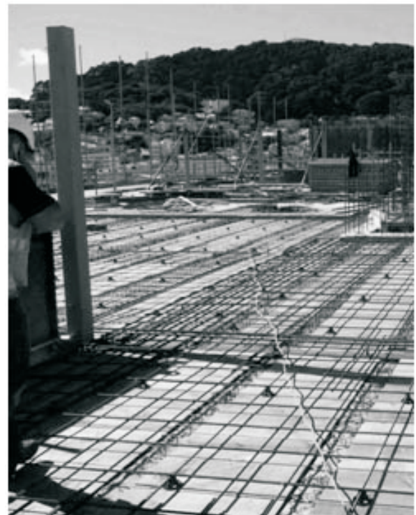
Fig. 3 Suspended floor slab ready to be poured. Note band of heavy diaphragm reinforcement to the left.
