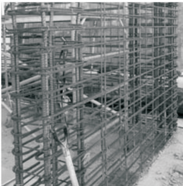
Fig. 1 Shear wall reinforcement towards top of building.
