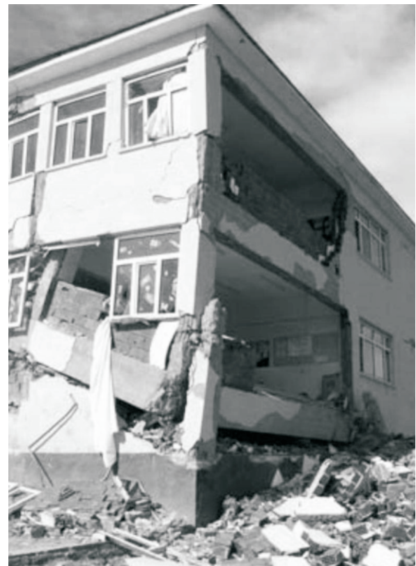
Fig. 6 Remains of the corner column of the ground floor of the building shown in Figure 5. The corner column failed in shear.
