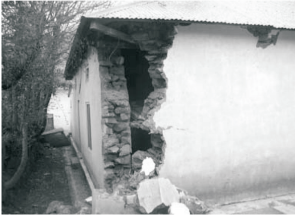
Fig. 6 Damaged corner of a building in Mazaffarabad.
