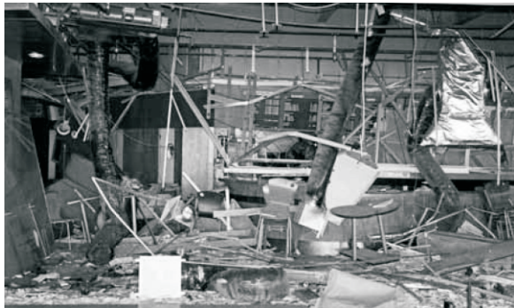
Fig. 10. Nonstructural damage at the Santiago International Airport terminal (photo: E. Miranda)
