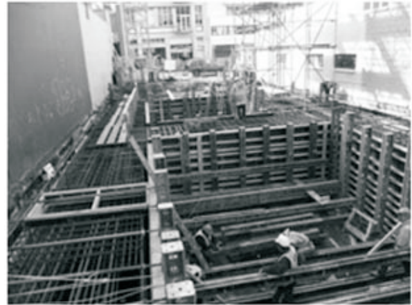
Fig. 2 Reinforcement and form work for the foundation beams.
