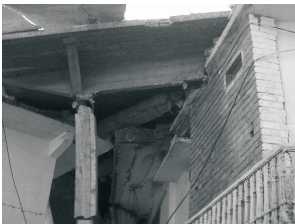
Fig. 4 Collapsed building due to strong beams and weak columns.
