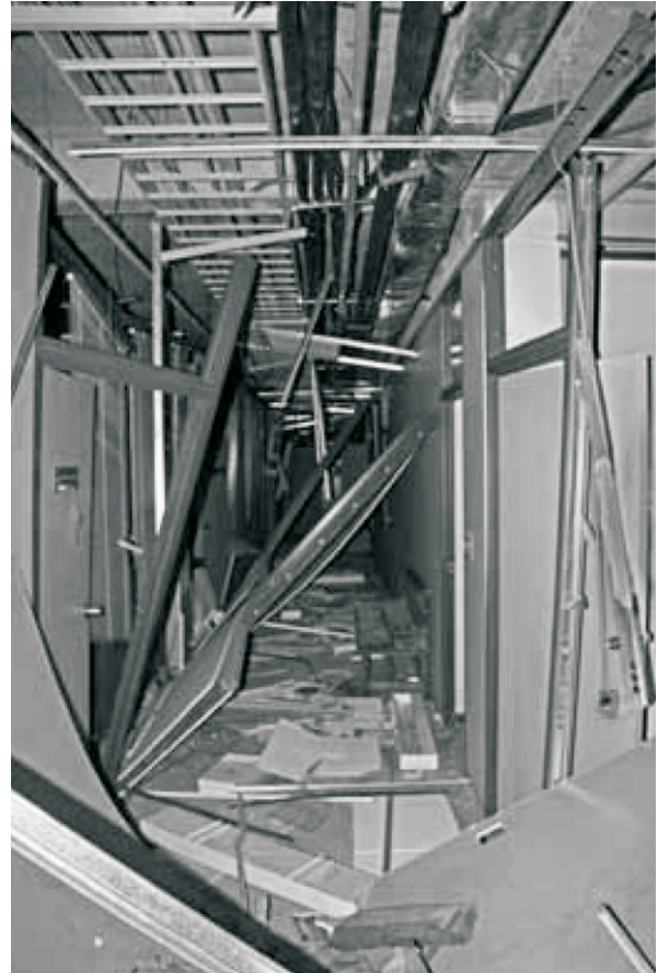
Fig. 9. Nonstructural damage in the Talca Supreme Court building constructed in 2003 (photo: E. Miranda)
