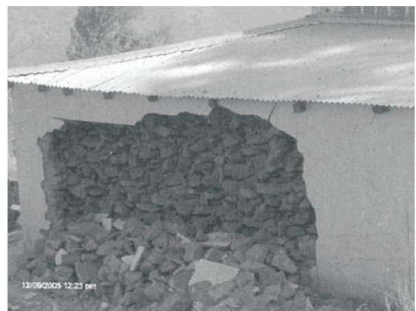
Fig. 7 Collapse of external veneer of stone masonry wall.
