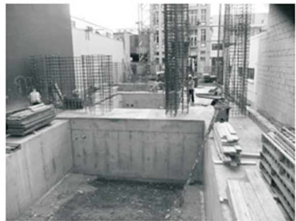
Fig. 3 Completed foundation beams with the shear wall reinforcement projecting above, to the left.
