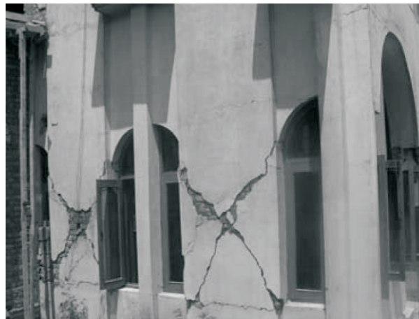
Fig. 5 Diagonal shear failures of masonry wall piers.
