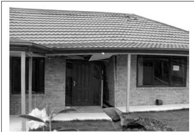
Fig.7. Above: Large lateral spreading like a rupture passed through the foundation near Courtenay Drive in Kaiapoi. Below: This house slid more than 1.2 m and tilted significantly (near Courtenay Drive in Kaiapoi) (photos: Lai).
