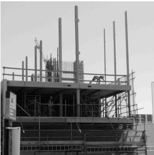
Fig.1. The superstructure under construction with transverse shear wall reinforcement and gravity-only steel columns.
