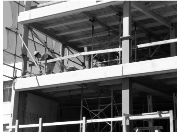
Fig.2. Suspended floors consist of primary steel beams carrying precast concrete planks with timber infills supporting 75 mm RC topping.
