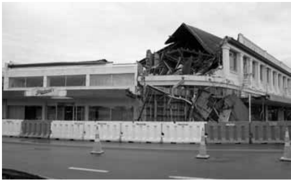
Fig.8. Blackwell's Department Store on William Street in Kaiapoi suffered extensive structural damage (photo: Arendt)
