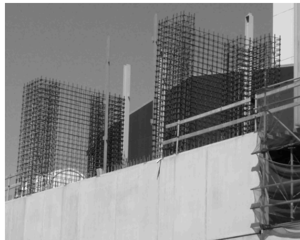
Fig.3. A longitudinal precast panel shear wall with the two transverse shear walls behind.
