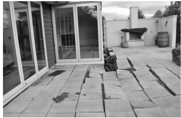
Fig. 6. Structures damaged by lateral spreading and post-liquefaction differential settlement. Above: Residential structure in Spencerville. Below: St. Paul's Church in Dallington.
