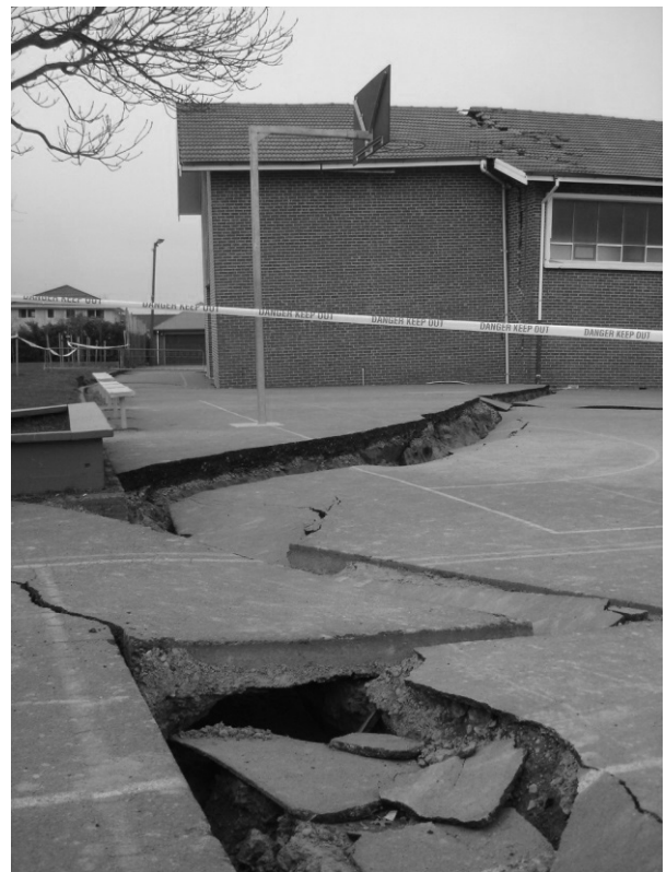
Fig. 6. Structures damaged by lateral spreading and post-liquefaction differential settlement. Above: Residential structure in Spencerville. Below: St. Paul's Church in Dallington.
