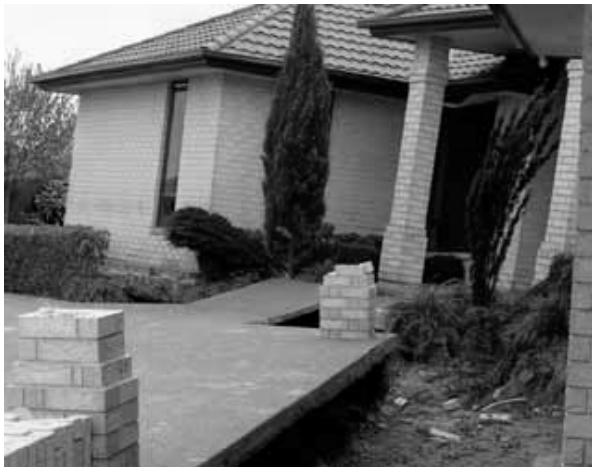
Fig.7. Above: Large lateral spreading like a rupture passed through the foundation near Courtenay Drive in Kaiapoi. Below: This house slid more than 1.2 m and tilted significantly (near Courtenay Drive in Kaiapoi) (photos: Lai).
