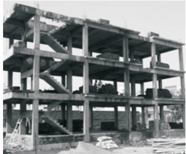
Fig. 2. Infill walls are about to be laid between frame members.
