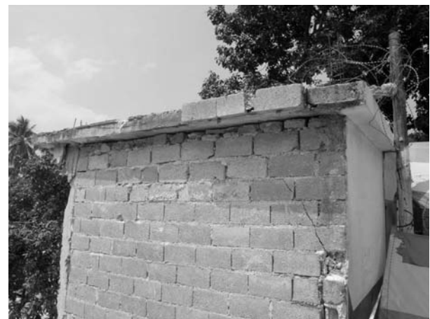
Fig. 8. Masonry walls are built short of the roof slab for all types of masonry construction; block debris is added to fill in the gap.
