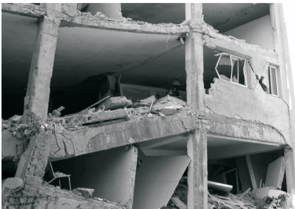
Fig. 11d. Complete failure of infill panels followed by partial collapse due to poorly confined columns.
