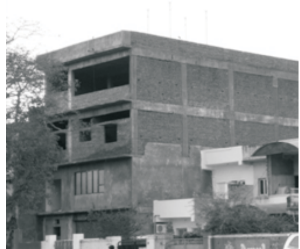
Fig. 3. If constructed of confined masonry, the longitudinal walls would provide excellent seismic resistance.
