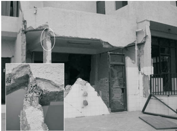
Fig. 11b. Damage to reinforced concrete beam-column joints following failure of masonry infill.
