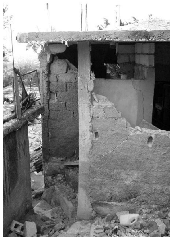
Fig. 10. Infilled frame construction is distinguishable by clean lines between columns and walls. Typical failure is out-of-plane toppling, as shown
