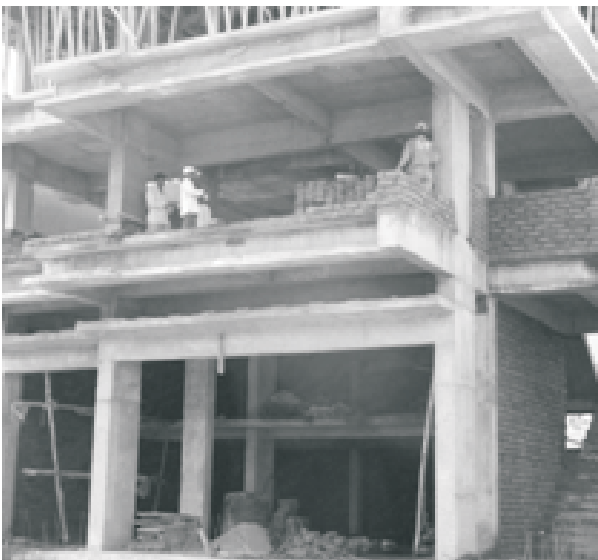
Fig. 1. Masonry infills under construction within the RC frames.
