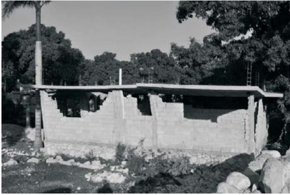
Fig. 11a. Typical failures of infill masonry construction: Infill wall failure initiated at openings resulting in large rotational demands at beam-column joint.
