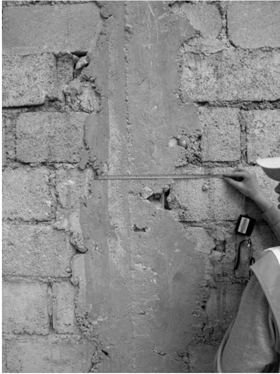
Fig. 9. Wall-first construction is identifiable by the oozing of the column concrete around the masonry blocks.
