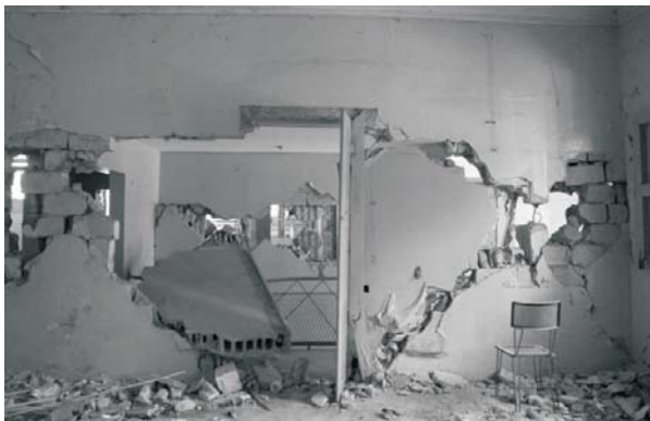
Fig. 11c. Common brittle in-plane shear failure (X-cracking) of masonry wall.
