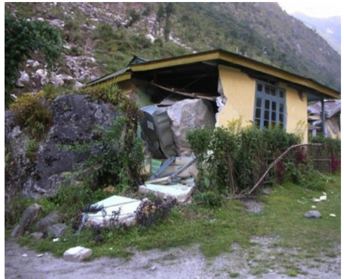
Fig. 4 Damage to houses due to rolling boulder at Lingzja and Chungthang (photos: Arun Menon and Rupen Goswami).
