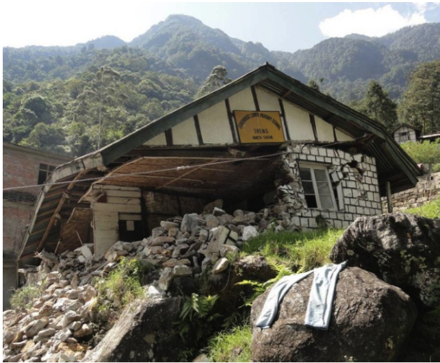
Fig. 7 Collapse of masonry building of the primary school at Tbeng (photo: Arvind Jaiswal).
