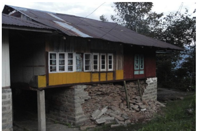
Fig. 5 above, Typical ekra house at Gangtok (photo: Alpa Sheth) below, typical house with wooden planks (Sbee Khim) with damaged rubble masonry plinth (photo: AR Vijayanarayanan).
