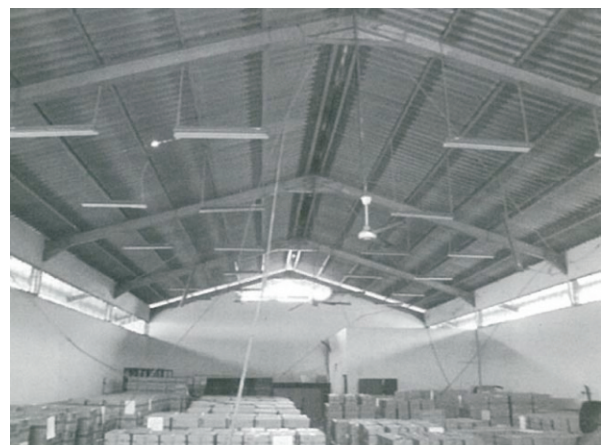
Fig. 5 Collapsed roof-level rod bracing in warehouse.
