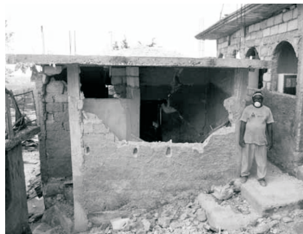
Fig. 9. Typical out-of-plane failure of an infill masonry construction (photo: Anna Lang).
