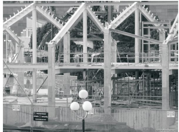
Fig. 2 Steel portal frames of the superstructure. They support a suspended reinforced concrete floor over a portion of their spans.
