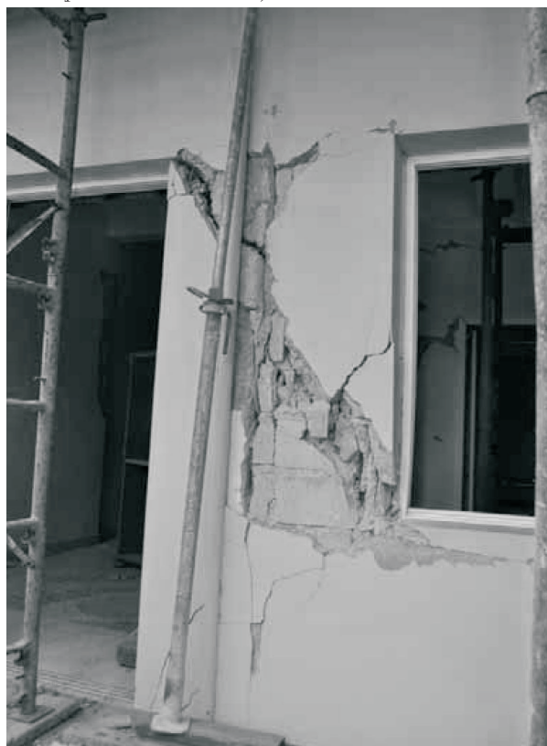
Fig. 7 Reinforced CMU wall from a hotel in Pentonville (photo: Amanda Lewis).
