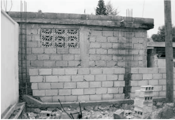
Fig. 10. In foreground, new wall under construction shows staggering of blocks within the column cavity; this mechanically locks the masonry wall to the columns, causing them to act as a unit. In background, a typical one-story CM residence (photo: Anna Lang).
