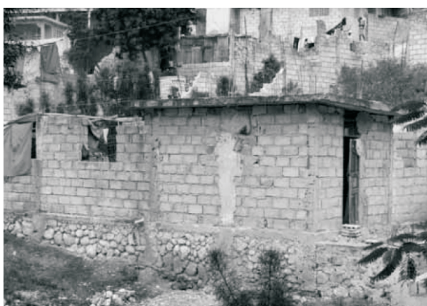
Fig. 8. Typical construction of a residence, showing a rock rubble foundation, confined masonry construction technique, and reinforced concrete slab. Note blocks added to the top of the walls and reinforcement emerging from the slab, ready for construction of another level (photo: Anna Lang).
