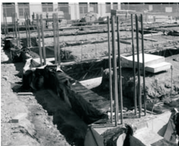
Fig.1 Foundation beams and reinforcing starters for columns. After the plastic sheeting under the beams has been protected by cheap sheet material and the excavation has been backfilled the sheeting is bent over and jointed to sheeting providing moisture resistance to the ground floor slab.
