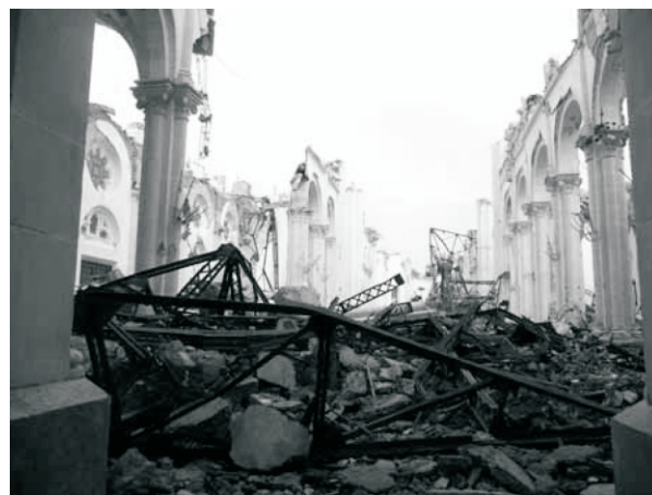
Fig. 6. Collapsed roof, interior of National Cathedral, Port-au-Prince (photo: Martin Hammer).
