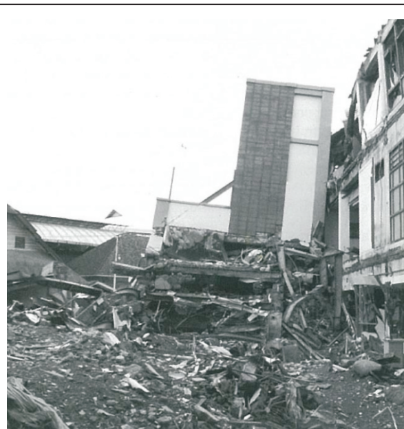
Fig. 4 Collapsed 5 level two-way steel MRF addition to hotel.
