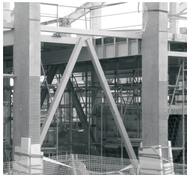
Fig. 3 One of several braced bays providing seismic resistance along the length of the building.
