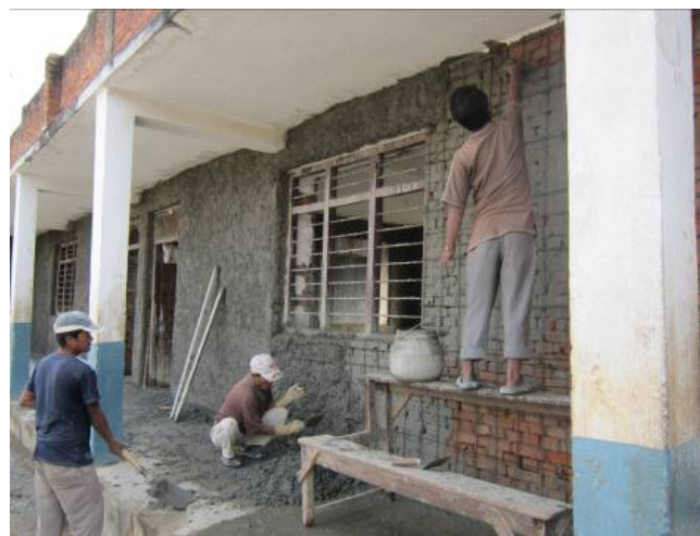
Fig. 12 Micro-concreting grouting.
