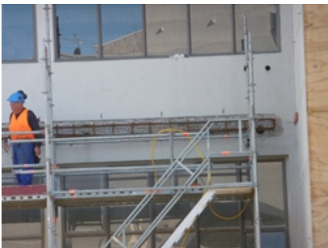
Fig. 2 Reinforcing tied into the existing building that will become the means of transferring seismic forces from the old into the new structure.
