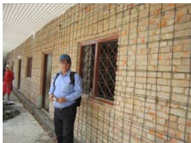
Fig. 8 RCC Jacketing of exterior walls.
