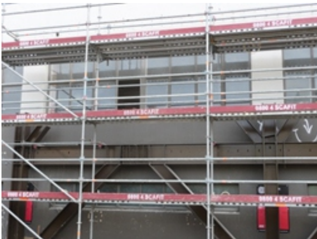
Fig. 1 The eccentrically braced frame with its beam at first floor.
