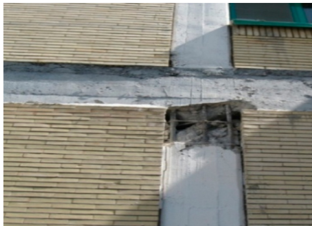
Fig. 6 Herris Hospital structural damage: plastic hinges in beam column joints (center) and diagonal crack in a column (bottom).
