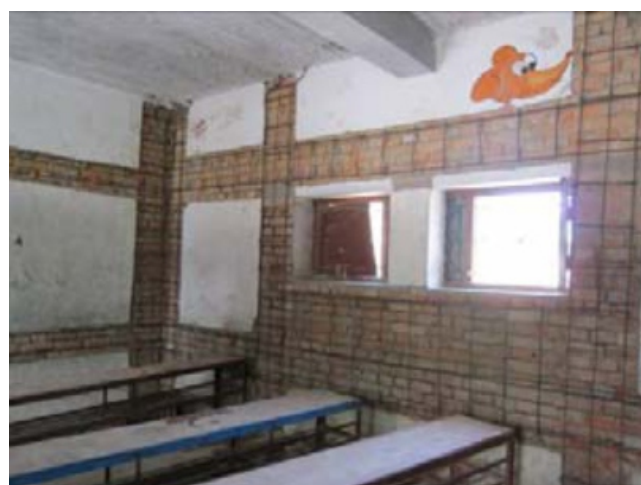
Fig. 9 RCC splints and bands on interior walls level.
