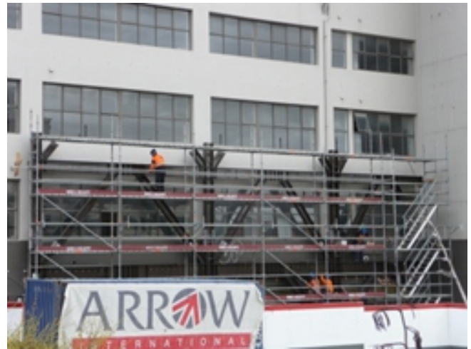
Fig. 3 The eccentric braced frame at the second storey level is being bolted to the steel framing beneath.
