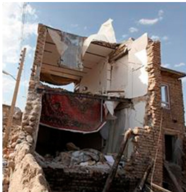
Fig. 4 Failure of heavy steel jack-arch and concrete roofs, and walls of unreinforced masonry buildings (photos: Mebr News Agency; Bastami).
