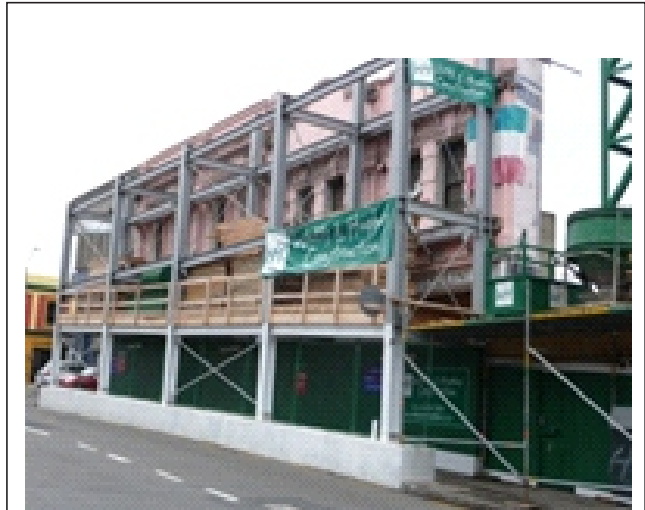
Fig. 1 Unreinforced masonry facade with its temporary restraining structure.
