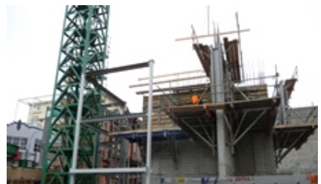
Fig. 3 New shear walls in each direction with the old facade behind.
