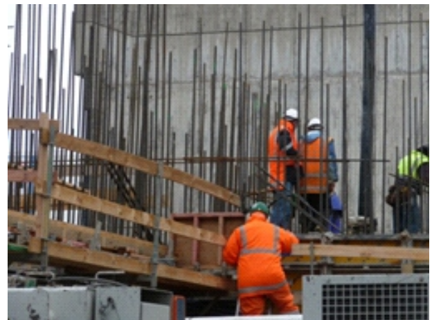
Fig. 2 Workers fix reinforcing steel for the new RC shear walls.
