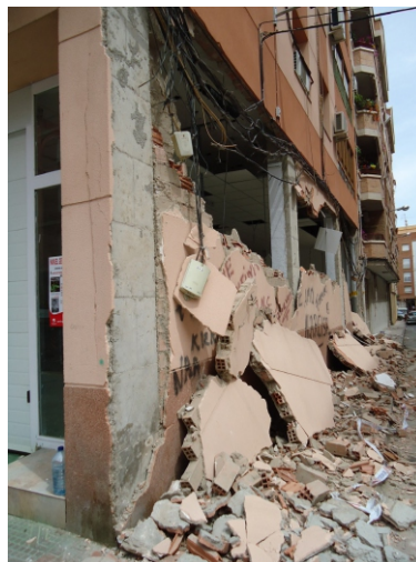
Fig. 9 Damaged masonry infill walls at ground floor.
