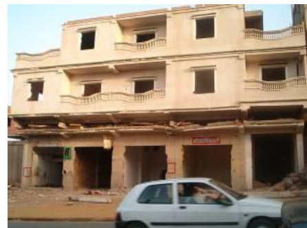
Fig. 7 Failure due to soft floor effect.
