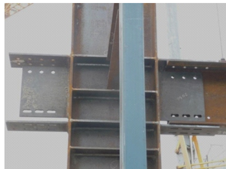
Fig. 4 Slotted holes in the bottom connections of the rigid joint for damage-avoidance design.
