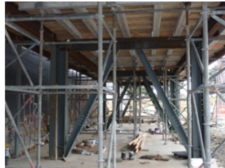
Fig. 2 The eccentrically braced frames resisting gravity and transverse loads.
