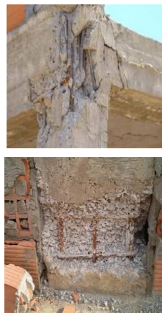
Fig. 5 Poor workmanship and bad quality concrete helped the seismic collapses.
