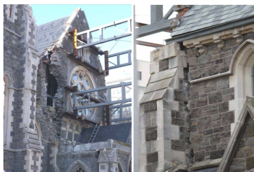
Fig. 11 Christchurch Anglican Cathedral: out-of-plane overturning of the front façade.
