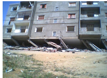
Fig. 6 Failure due to short column behaviour.
