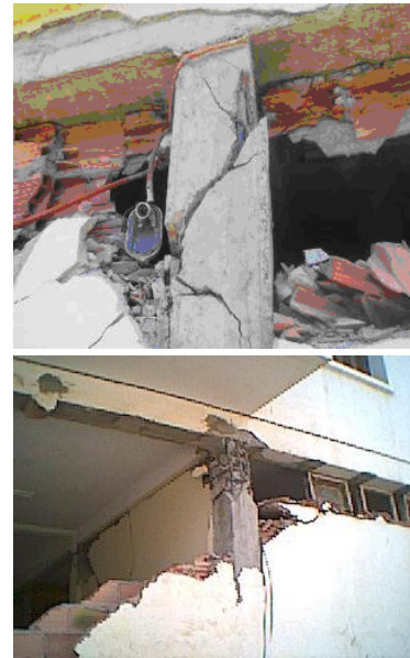
Fig. 6 Failure due to short column behaviour.
