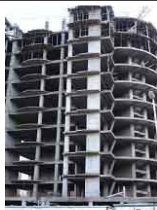
Fig. 9 Buildings with combined shearwalls/ beam-column framed structure under construction at the time of the 2003 earthquake – no sign of distress was shown.
