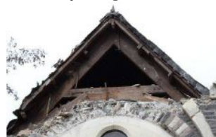
Fig. 13 Overturning of the front façade gable.
