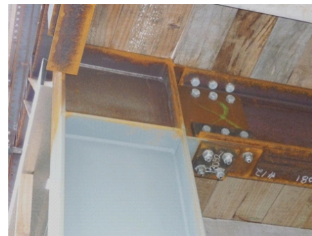
Fig. 3 A beam-column rigid joint in the moment frame.
