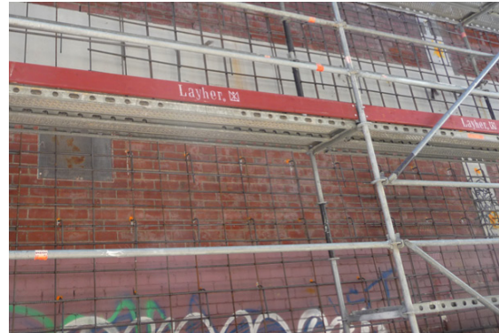
Fig. 1 The rear wall of the building and the reinforcing cage for a new concrete wall.
