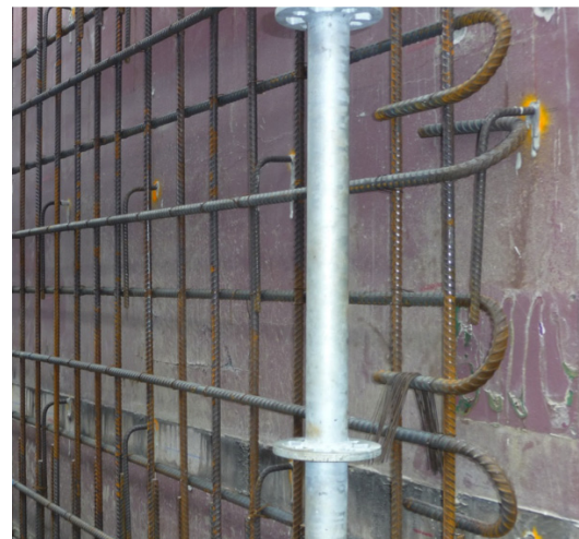
Fig. 2 Grouted-in bars, bent into the wall thickness, provide the temporary attachment points for the wall reinforcing and strongly connect new construction to the old.
