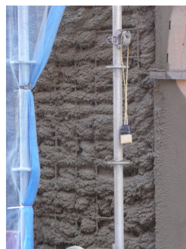
Fig. 3 The concrete has just been applied. It is trowelled over to form a smooth finish.
