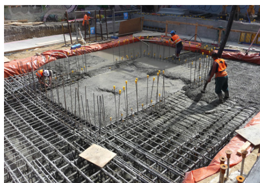
Fig. 3 Concreting of the foundation beams/raft under the structural core walls.
