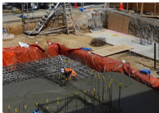
Fig. 2 The deep foundation beams under and outside the core, and perimeter pile reinforcing in the background.
