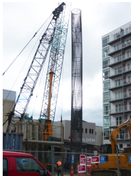
Fig. 1 A pile reinforcing cage with its welded spiral hoops to confine the concrete.
