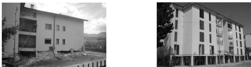
Fig. 6: Two recent examples of severe damage attributed to the soft first story irregularity in L'Aquila earthquake, Italy in 2009, (Photos, left: Holly Razzano, Degenkolb) and in Lorca, Spain in 2011.
