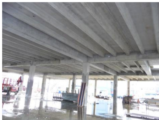
Fig. 1 The ground floor reinforced concrete structure consisting of two-way moment frames supporting precast concrete flooring.
