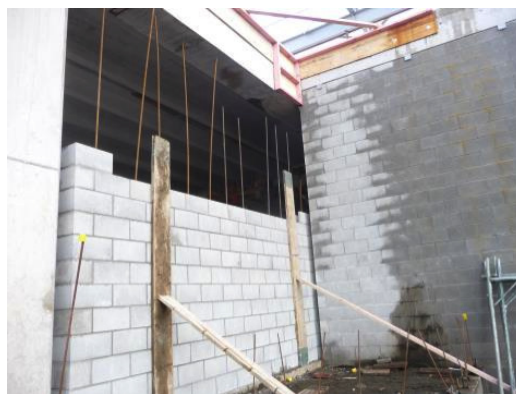
Fig. 2 A non-structural reinforced concrete masonry wall under construction. Vertical seismic separation joints are provided at each end of the wall.
