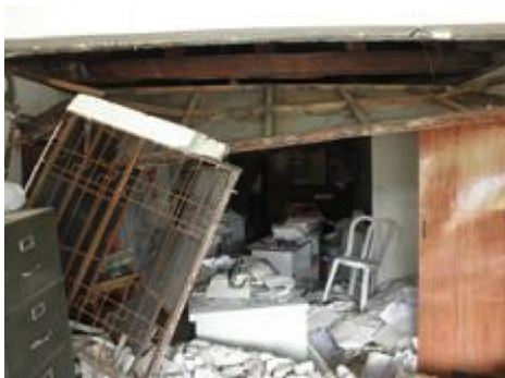
Figure 12. Examples of improper fixing of ceiling boards: (Left) Sagbayan Municipal Building, (Right) Market Building in Loon.
