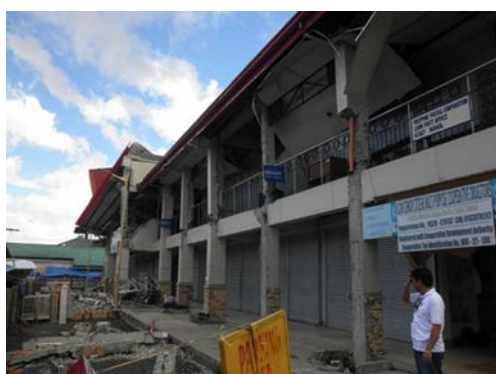
Figure 7. Examples of improper rebar works in Market Building in Loon: (Left) Heavy damage at the bottom of most of columns, (Right) Detail of the damage.
