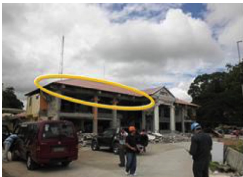
Figure 1. Municipal building of Sagbayan, Bohol. (Left): Heavy damage to partition walls and other elements, and (Right): inside the buildings.
