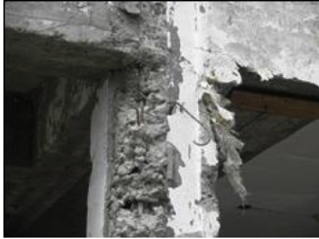
Figure 9. Examples of improper concrete placing: (left) Market Building in Loon, (Right) Sagbayan Municipal Office.
