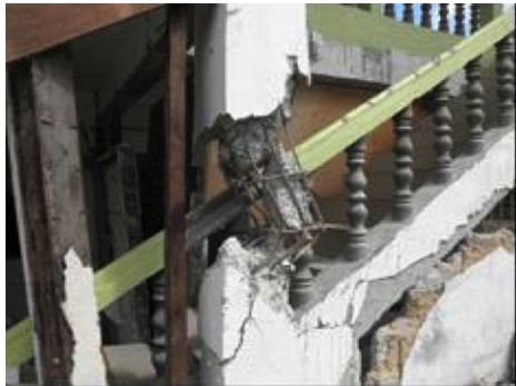
Figure 10. Examples of improper rebar works: (left) Barangay Office in Antequera, (Right) A building under construction, Basesy National High School.
