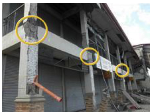
Figure 8. An example of improper rebar works in Market Building in Loon: (Left) Failures at panels, (Right) Detail of damaged part.
