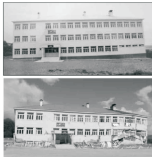
Fig. 12 Three story reinforced concrete moment-frame template school building with captive columns in Bingol before and after the may 1, 2003 Bingol earthquake.
