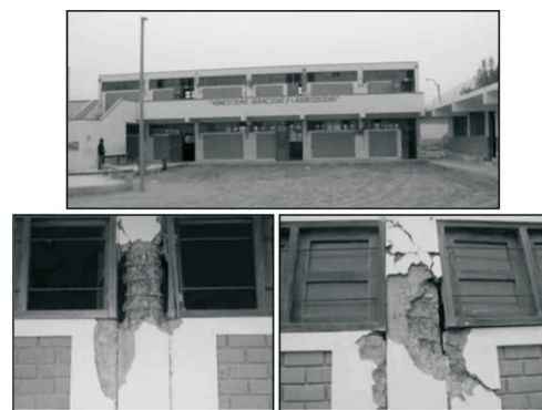
Fig. 18 Template school building designed according to 1977 code after 2001 Atico earthquake: (lower left) ground story column; (lower right) second story column
