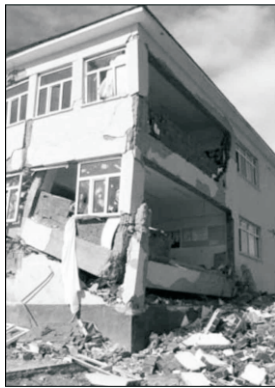
Fig. 13 Another view of collapsed school building. Note Column failure near beam joint.
