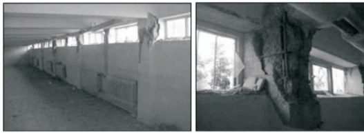
Fig. 11. View of dual system reinforced concrete template school building in Duzce after November 12, 1999 Duzce Earthquake. Captive exterior columns in basement failed.
