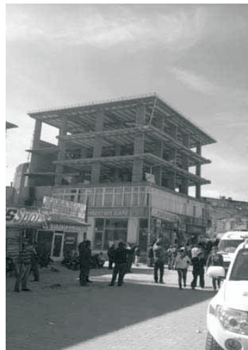
Fig. 5 Weak storey and asmolten slab
