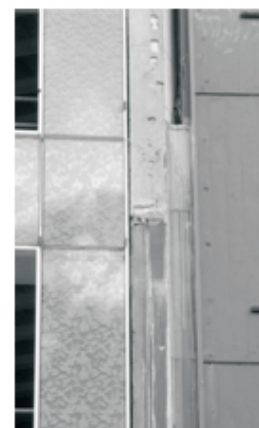
Fig. 4 The seismic gap between two buildings. The upper section of flashing has yet to be installed.
