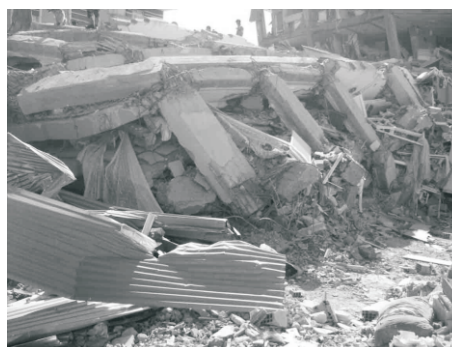
Fig. 7 Example of a collapsed RC frame building
