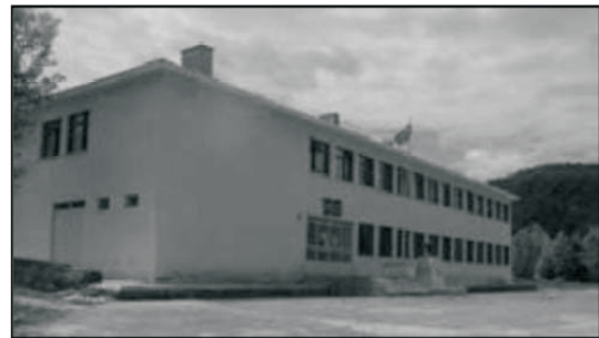
Fig. 10 Two-storey template reinforced concrete dual system school building in Kaynasli near Duzce. Building did not sustain structural or nonstructural damage during august 17,1999 and November 12, 1999 Duzce earthquakes.
