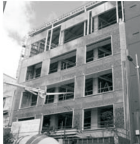
Fig. 1 Façade panels under erection with structural frame behind.
