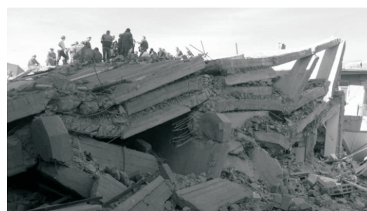
Fig. 8 Weak storey example
