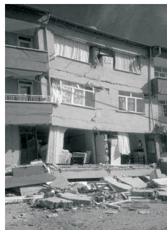
Fig. 6 Ground floor destroyed
