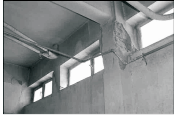
Fig. 15 Captive Column condition due to adjacent infill walls providing sufficient restraint in their out of plane direction.
